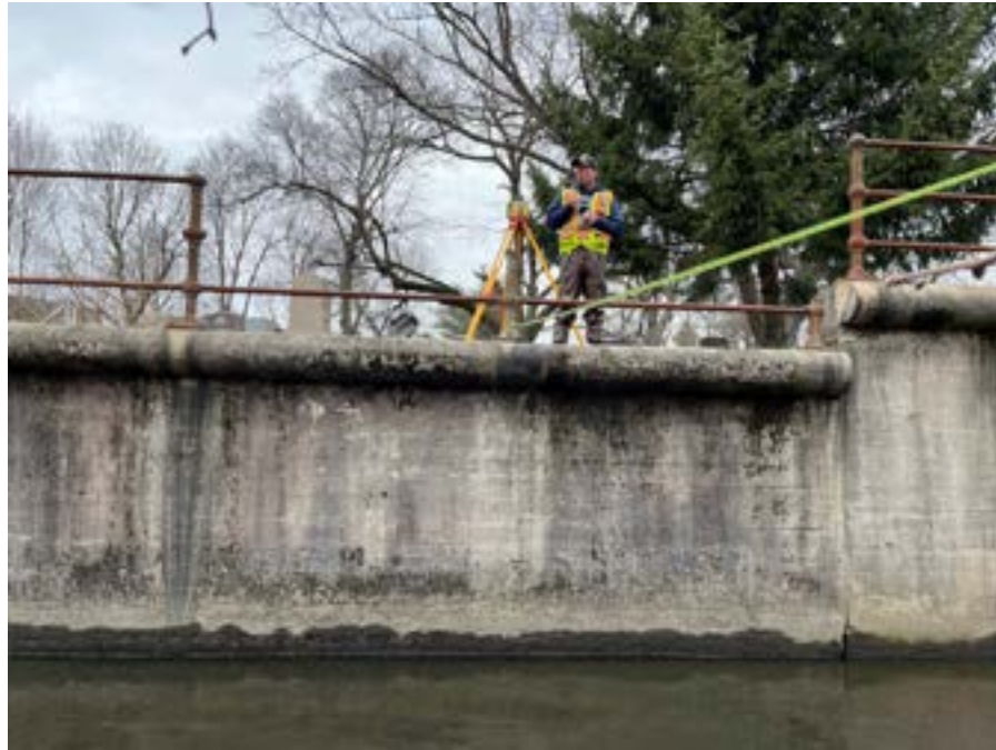
Photo 41. XS3 (Stream Segment 4) looking toward left bank.
