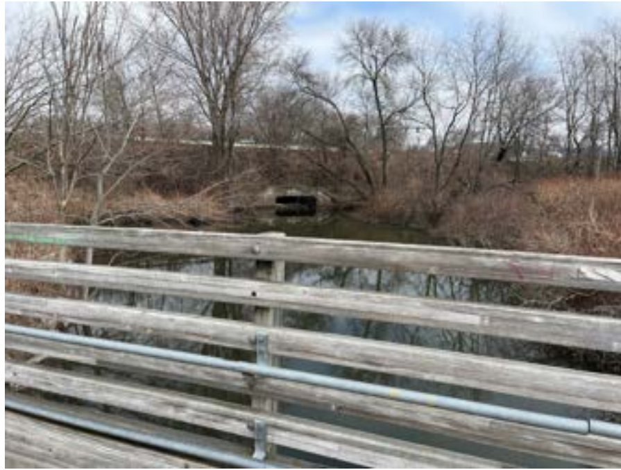
Photo 5. Looking downstream from Alewife Station Access Road toward Concord Turnpike.
