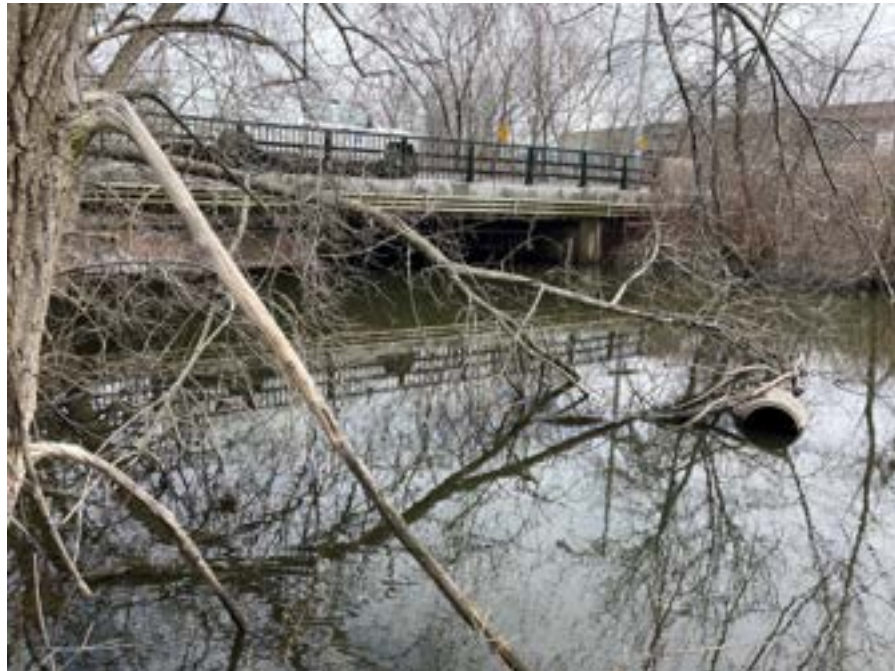
Photo 4. Looking upstream at Alewife Station Access Road crossing structure.
