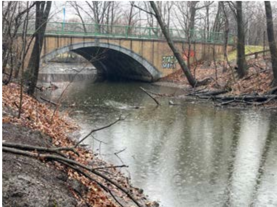
Photo 28. Looking downstream toward Mystic Valley Parkway inlet of crossing structure.
