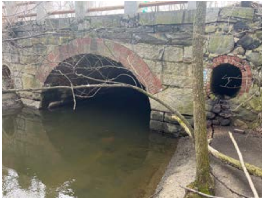
Photo 13. Massachusetts Avenue outlet of crossing structure.
