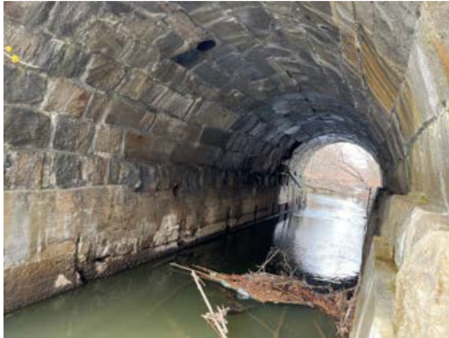
Photo 25. Looking downstream through Broadway crossing structure.
