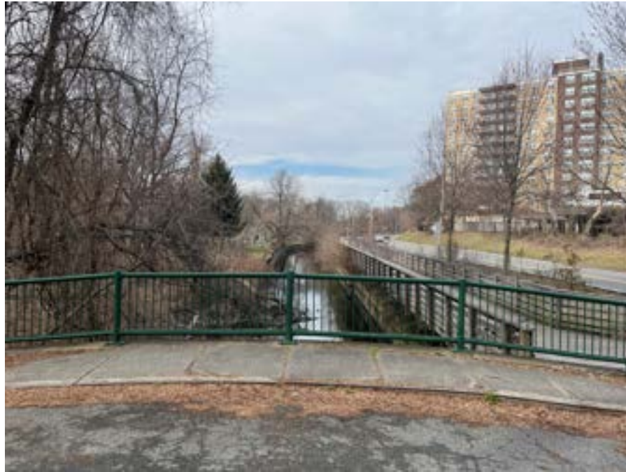
Photo 21. Looking downstream from Henderson Bridge at Stream Segment 4.
