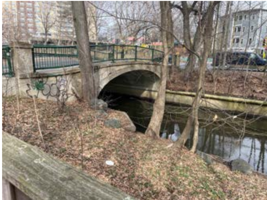
Photo 18. Henderson Bridge inlet of crossing structure.
