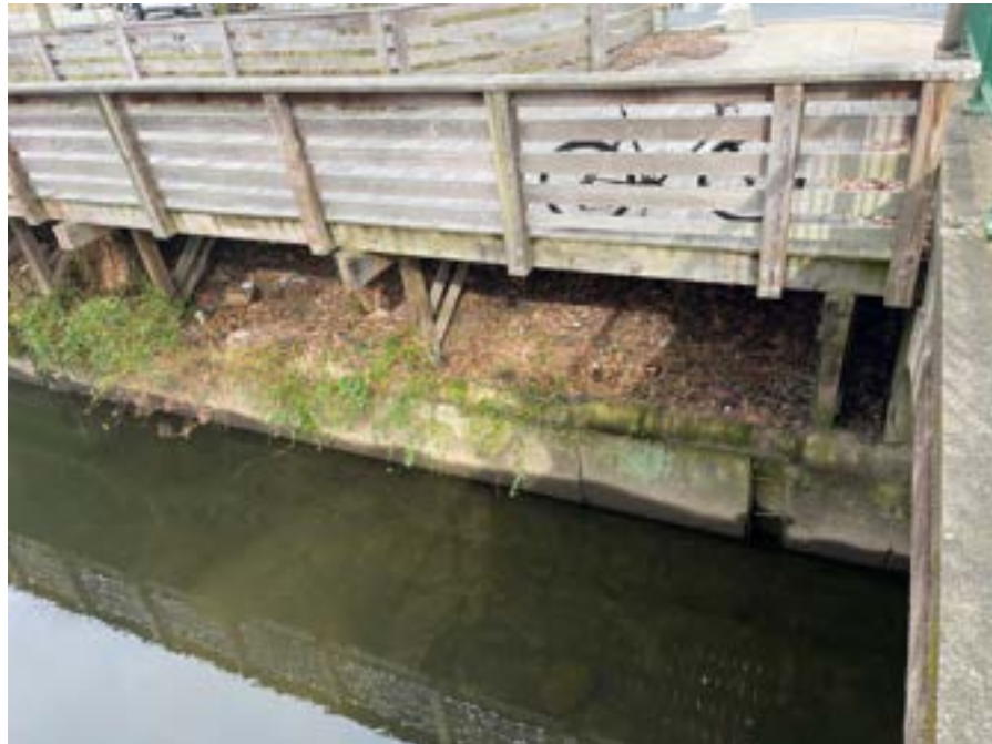
Photo 20. Henderson Bridge outlet of crossing structure.
