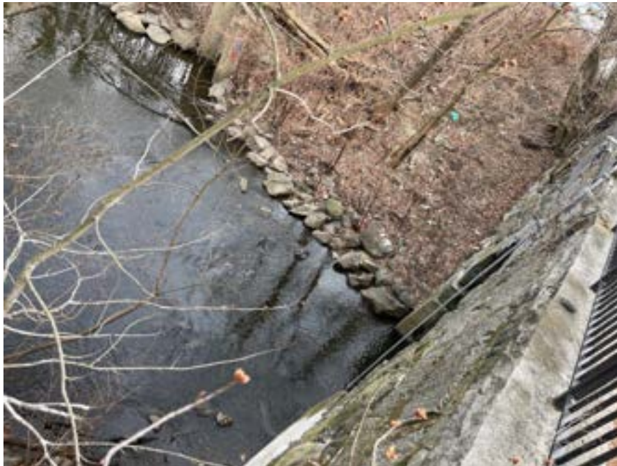
Photo 26. Broadway outlet of crossing structure.
