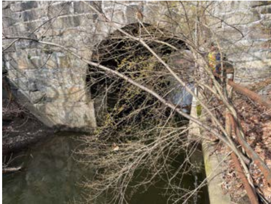
Photo 23. Broadway inlet of crossing structure.
