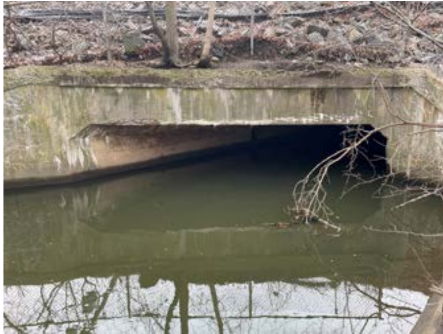
Photo 9. Concord Turnpike outlet of crossing structure.
