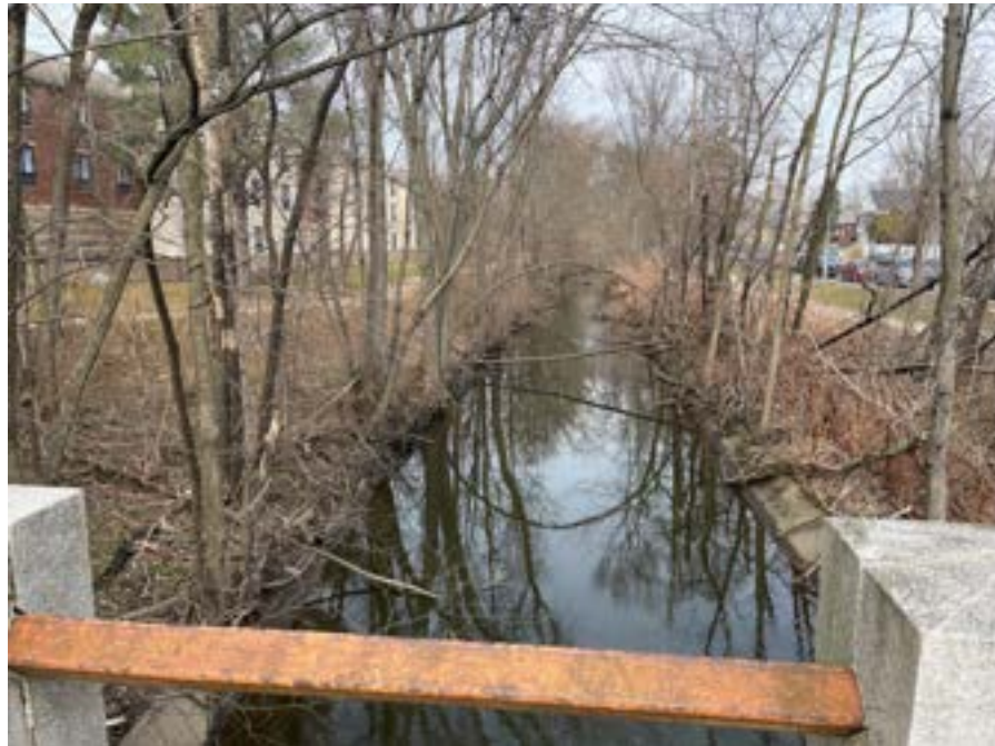
Photo 16. Looking downstream from Massachusetts Avenue at Stream Segment 3.
