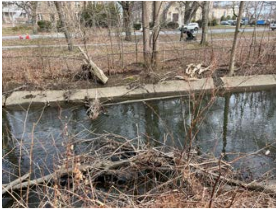
Photo 17. Typical debris jam in Stream Segment 3.
