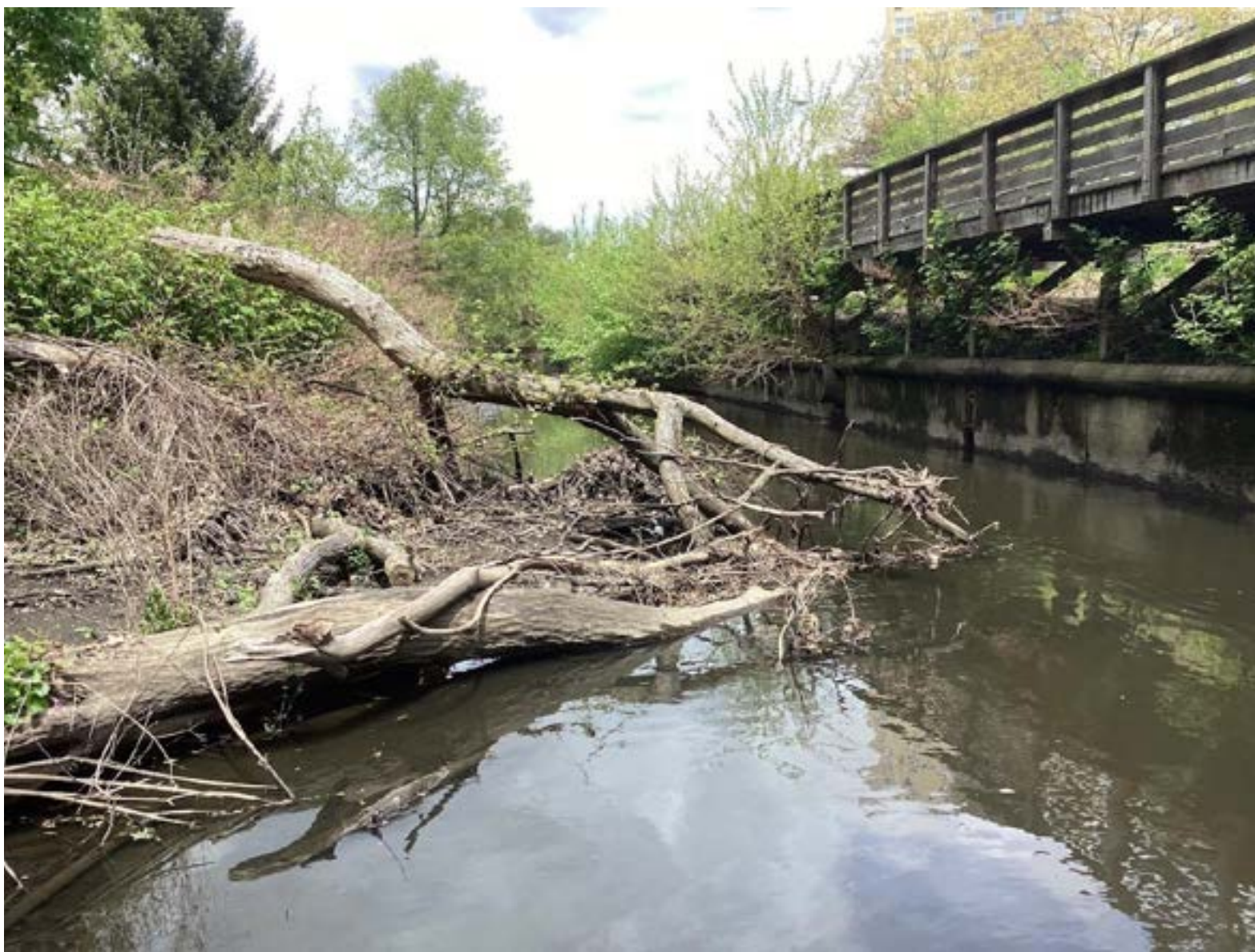
Figure 12. Reach C. Looking downstream with a large downed tree and log jam river left and the elevated boardwalk along Alewife Brook Parkway in the top right.
