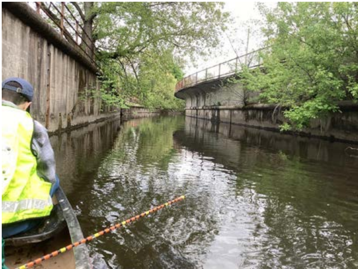
Figure 8. Sub-reach C, looking downstream with concrete lined walss on either side of the channel. St Pauls cemetery above on river left.
