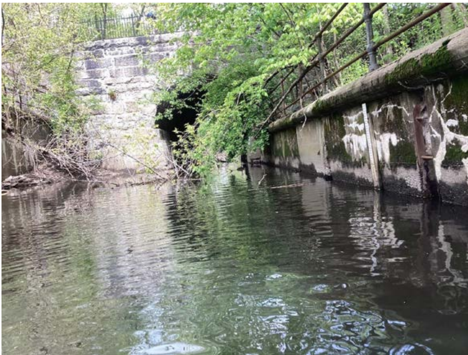
Figure 15. Reach C. Looking downstream towards the bridge at Broadway. Concrete walls line both sides of the channel throughout most of Reach C.
