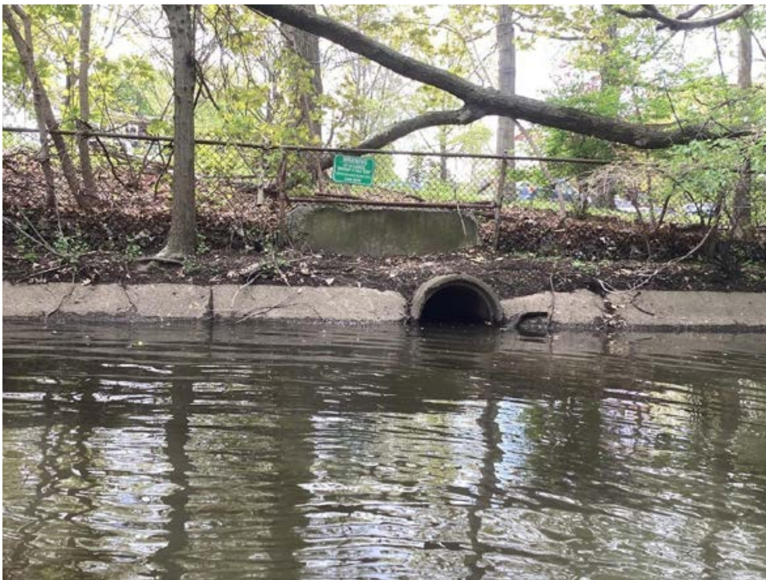
Figure 4. Reach A. Combined Sewer Outflow (CSO) CAM401B just upstream of Massachusetts Ave.
