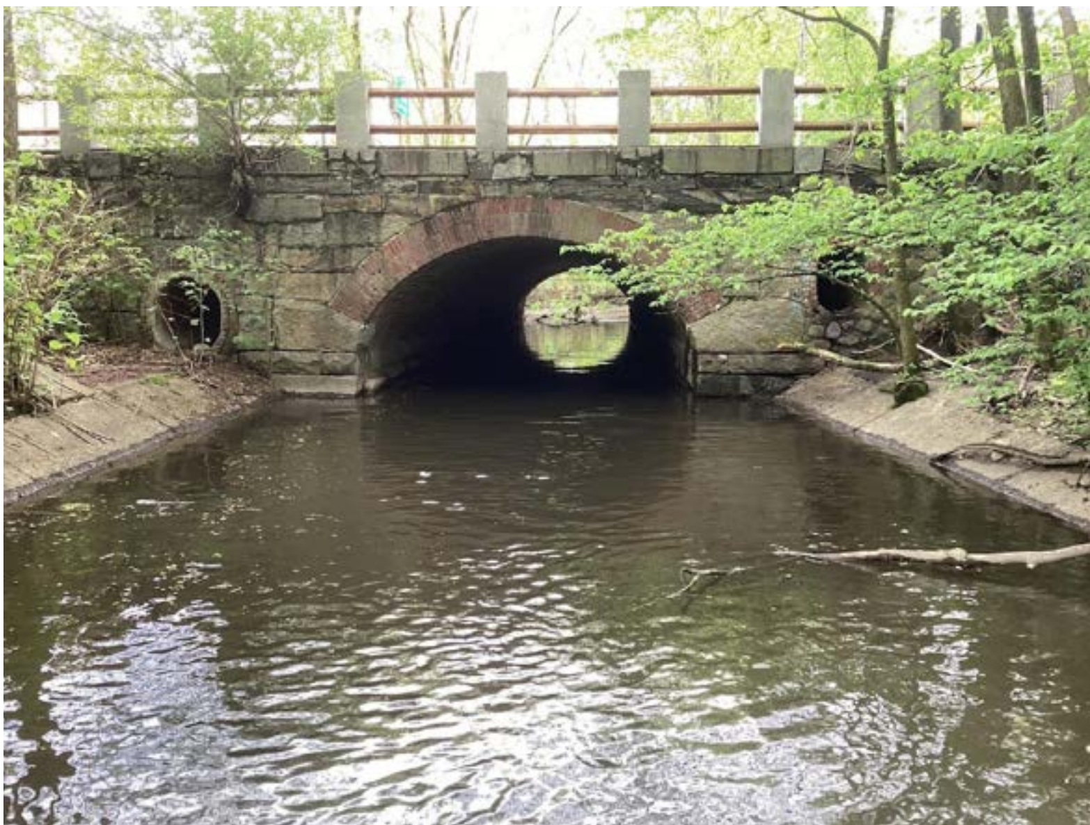
Figure 5. Reach A. Looking downstream at the Massachusetts Ave. bridge.
